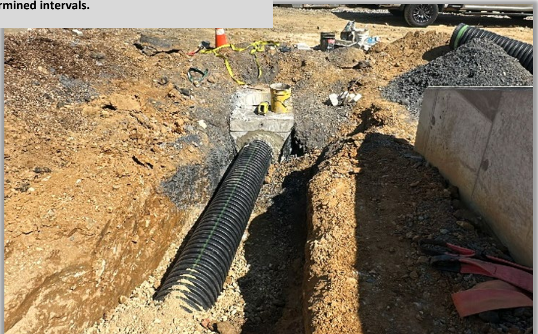
Storm Sewer Work Resumed to the West of the Family Center Wing. CHA coordinates with the Borough of Fountain Hill for monitoring of connections to public utilities.
