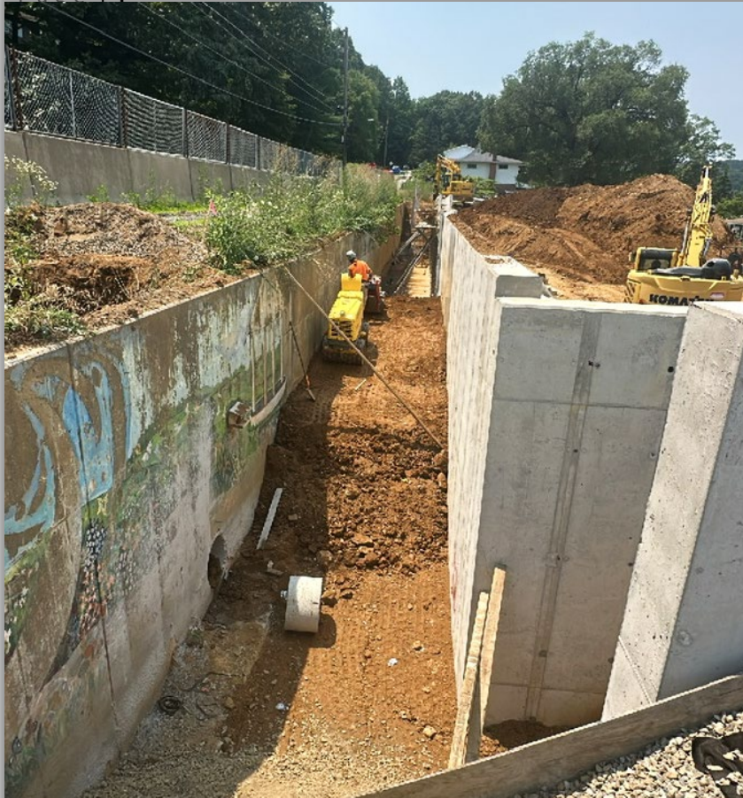
Backfilling and Compaction Activities Behind the Site Retaining Wall Along Moravia Street. Compaction behind the wall is critical to provide structural stability. Third party testing is used to verify successful compaction at pre-determined intervals.
