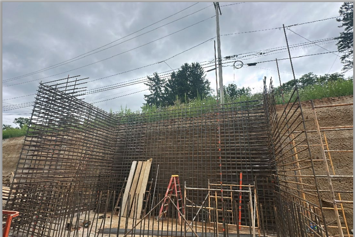
Installation of Foundation Wall Rebar for the Pedestrian Bridge.
