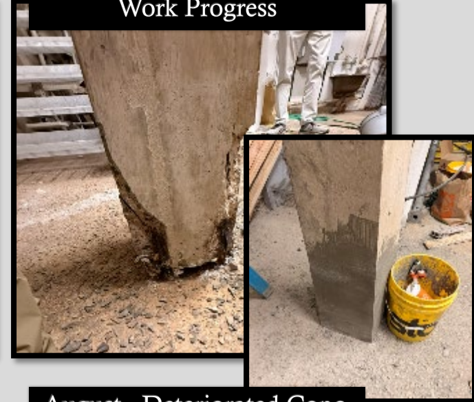
August - Deteriorated Conc. Work Progress
