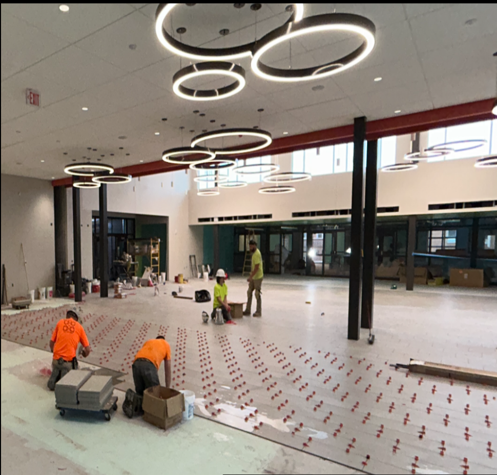
Cafeteria Ceramic Floor Tile Installation
