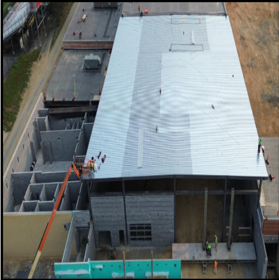
Gyn Extension Roof Decking
