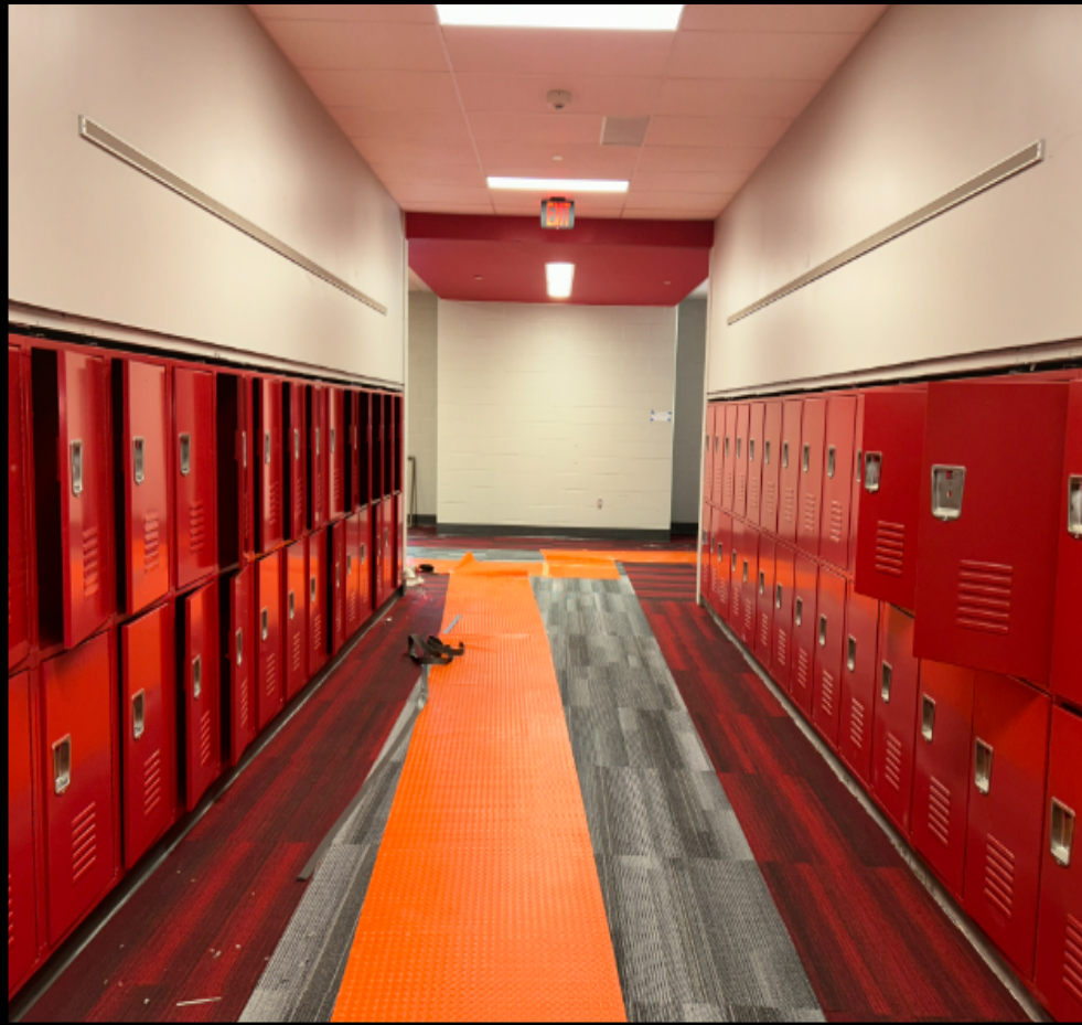
New Addition – 2 nd Floor Corridor
