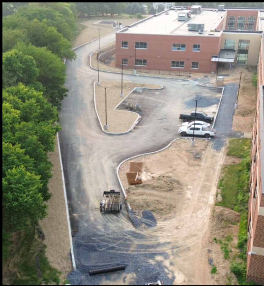
North Parking and ADA Bus Loop
