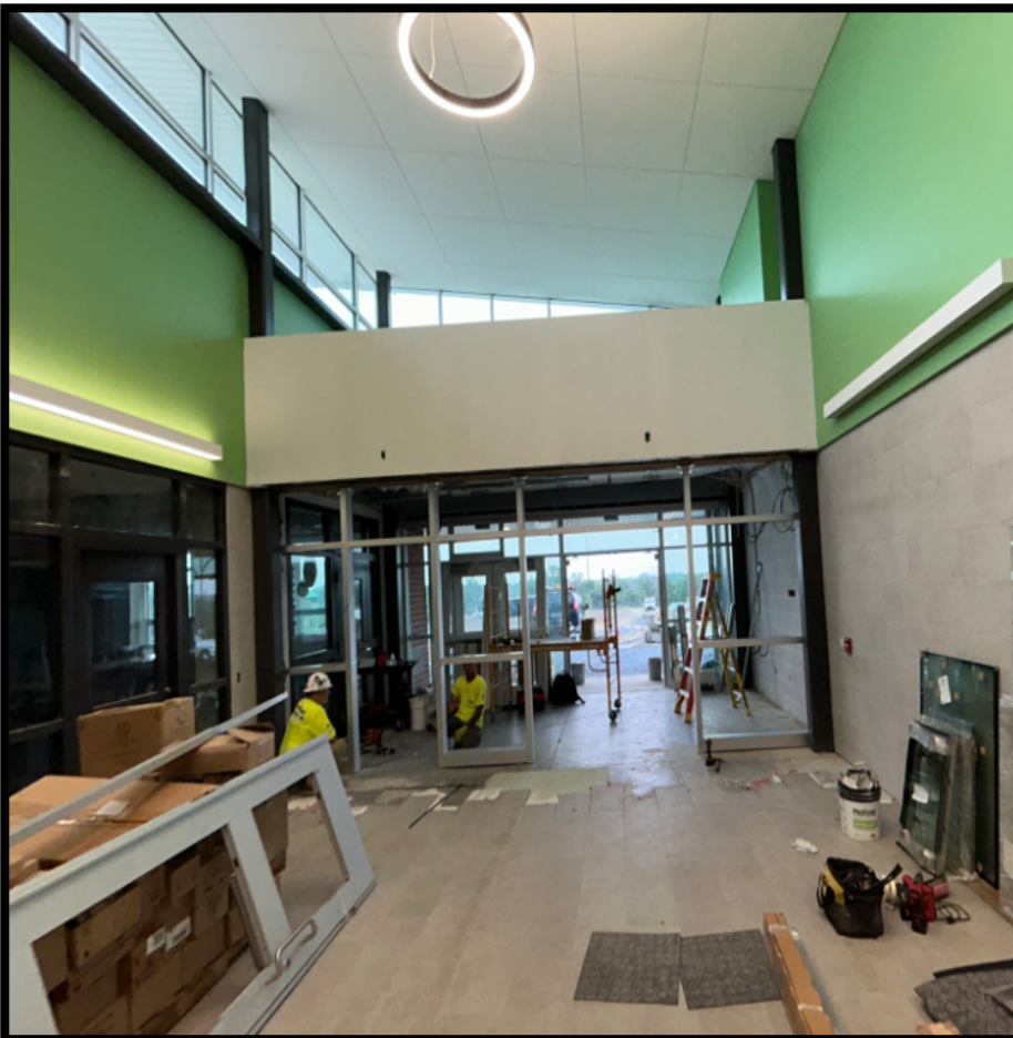
Main Street – Entry Door Installation
