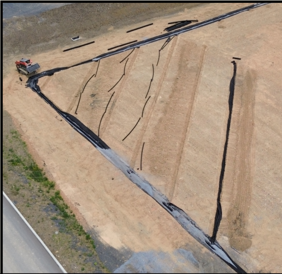
Athletic Field Under Drains Installation
