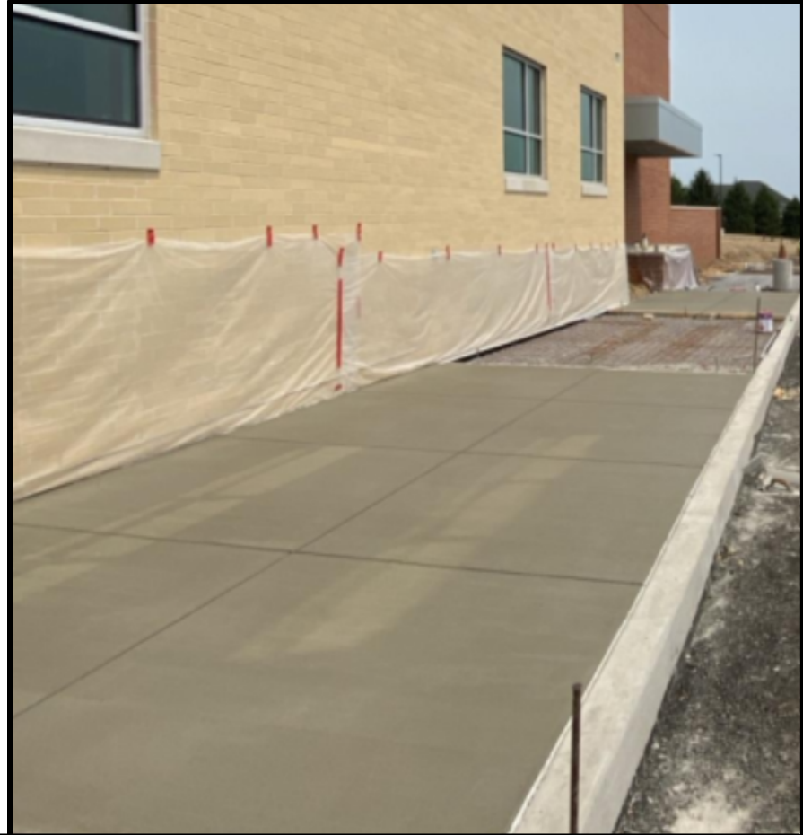
Sidewalk Installation Along Bus Loop
