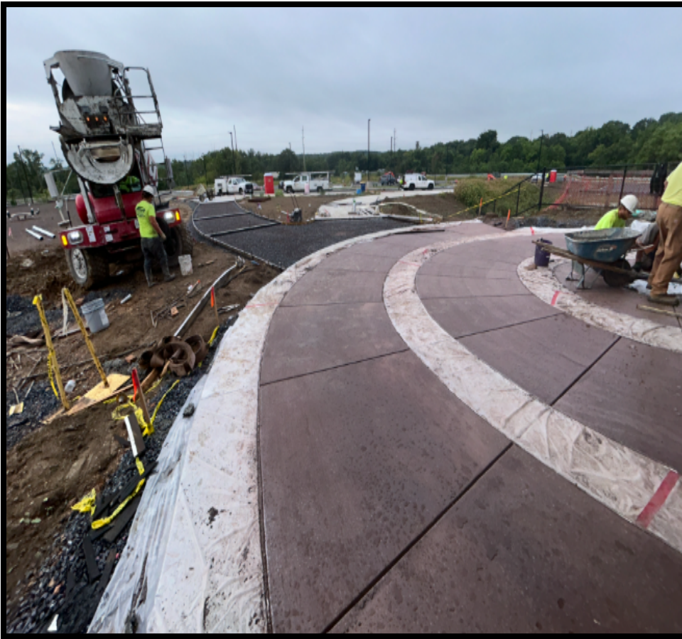
Placement of New Main Entry Accent Concrete
