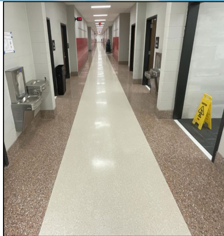
New Addition – 1 st Floor Terrazzo Flooring
