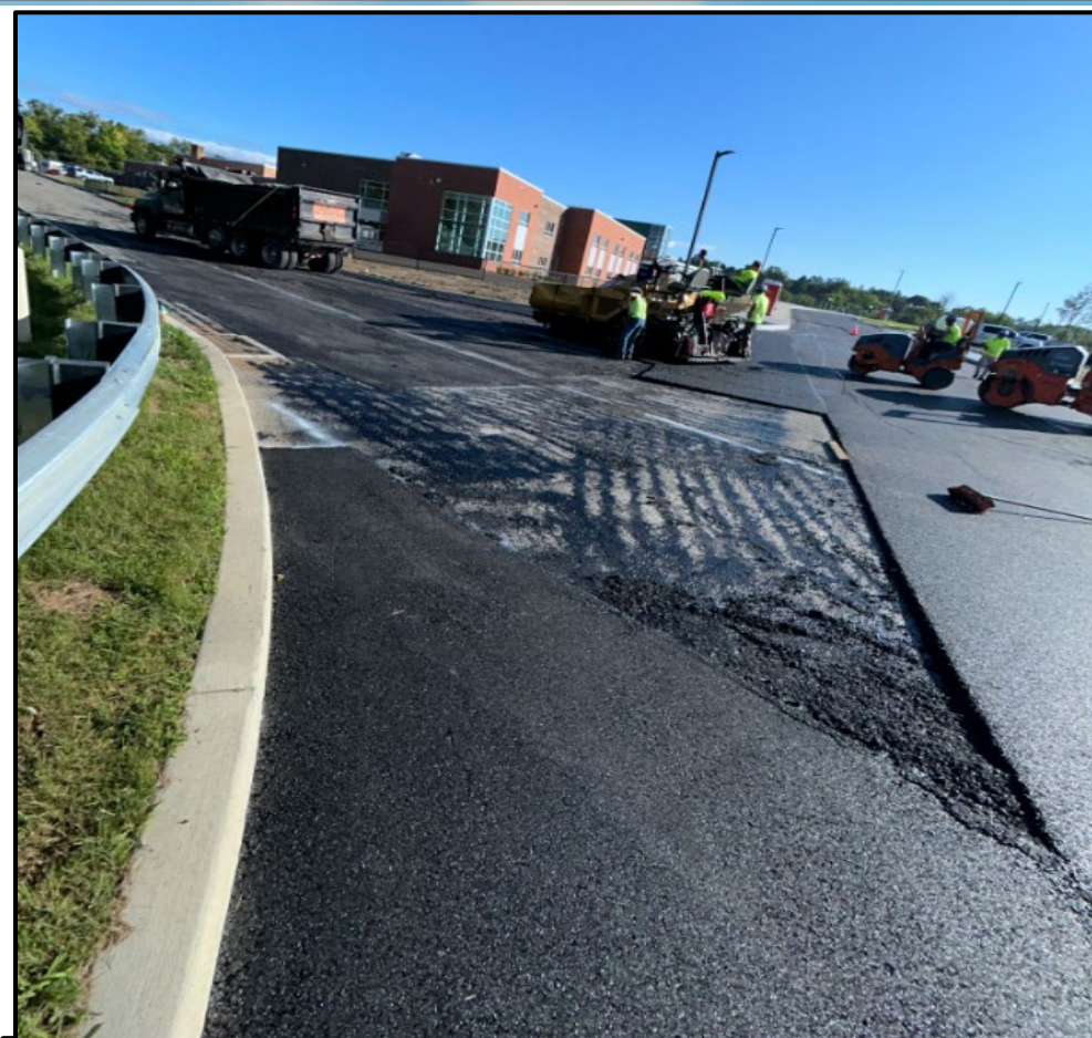
Final Asphalt Paving of Parking Areas
