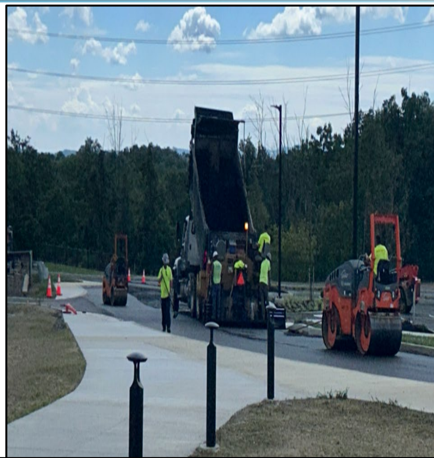
Final Asphalt Paving of the Bus Loop
