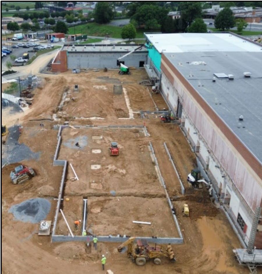
New Admin. Foundation/CMU Work
