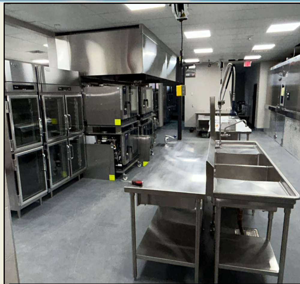
Kitchen - Cooking/Freezer Area
