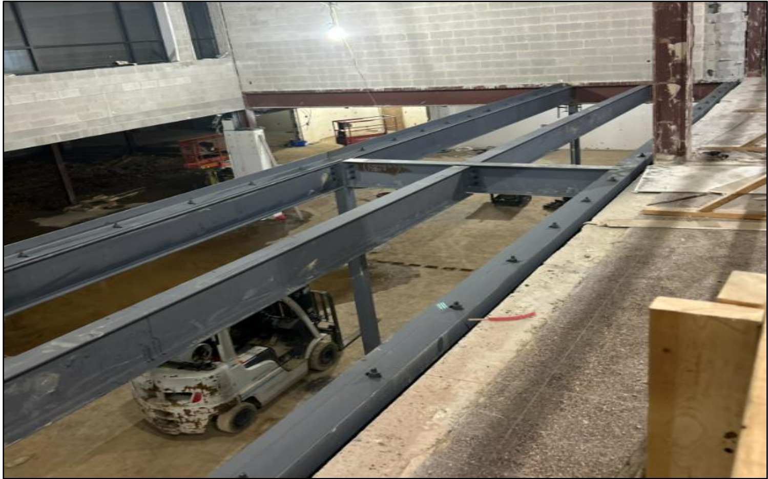
Second Floor Steel Installation for Media Center
