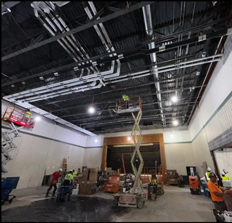
Ceiling Reno Work in Gym
