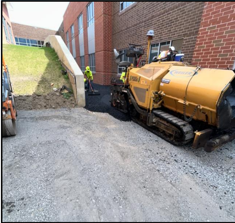
Final Asphalt Paving Between The Cafeteria and the New Addition
