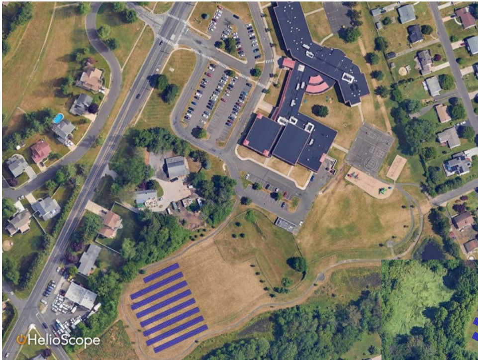
Cornwells Elementary Ground 401 kW (4%)
