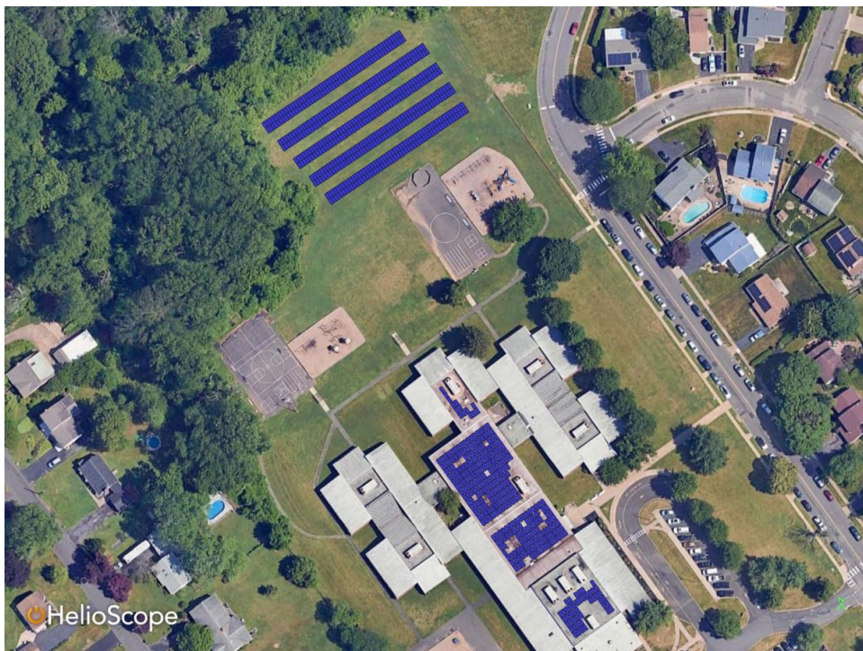
Belmont Elementary Ground 322 kW (3%)
